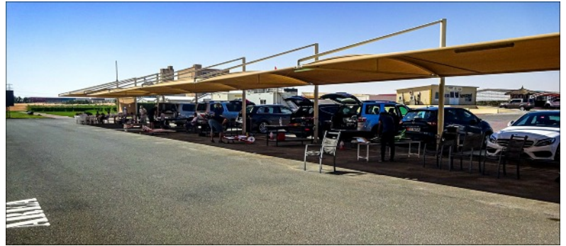
Shaded Parking right in front of the Pits Area
